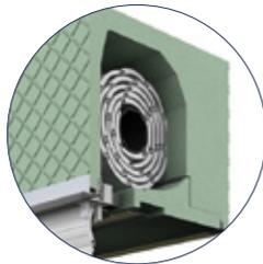
Maintenance of roller shutters based on the Roka-Top 2 RG system is possible only from the outside.
